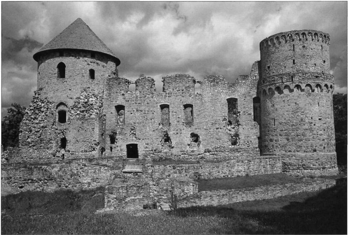
ABOVE The south face of the ruins of Wenden (Cesis), the headquarters of the Swordbrothers and for many years the headquarters of the Livonian Branch of the Teutonic Knights. On the left is the West Tower, which has a square cross section in its lower half and a circular artillery tower on top. On the right is the so-called 'Lange Hermann' tower.
